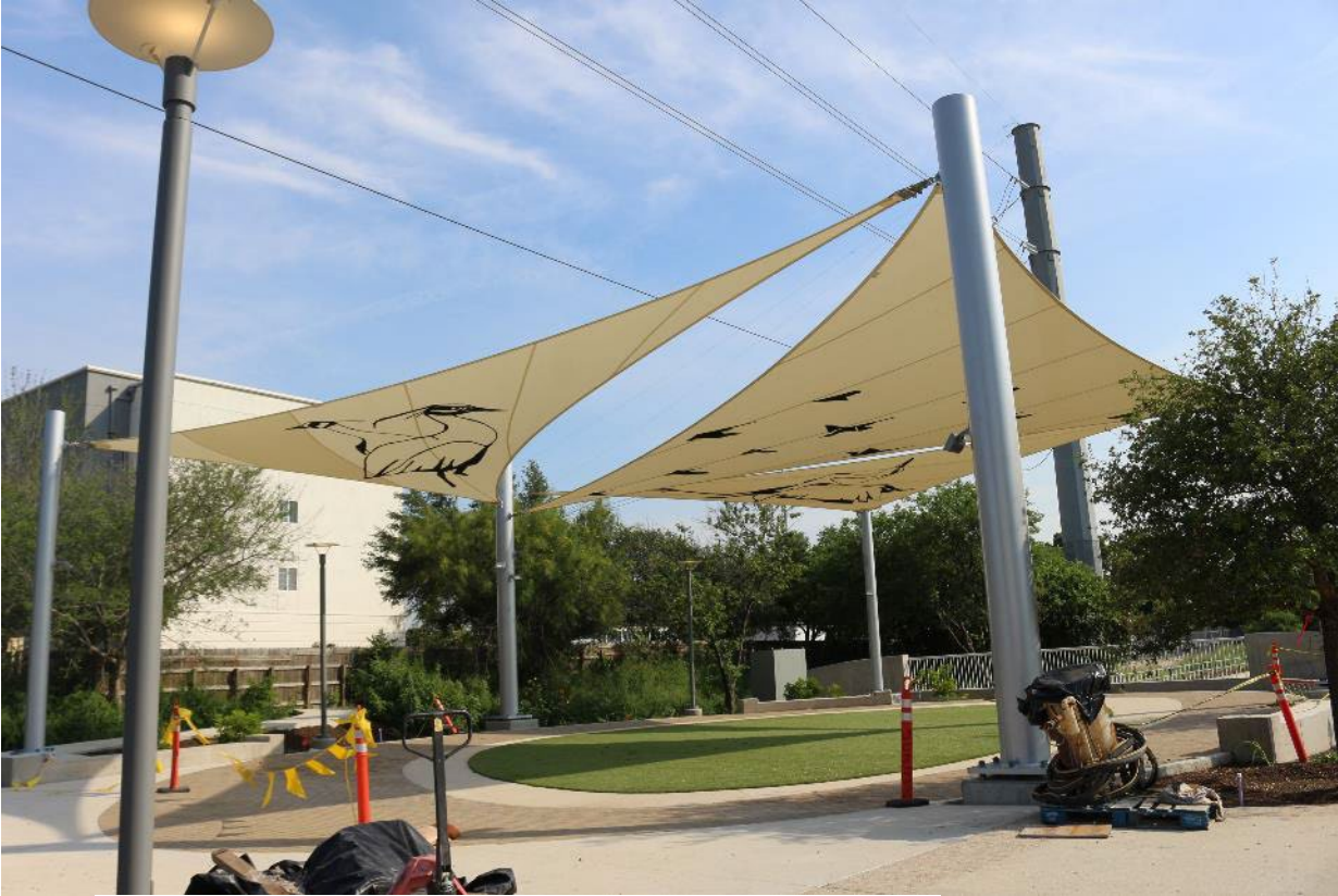
The shade structure has been installed.
