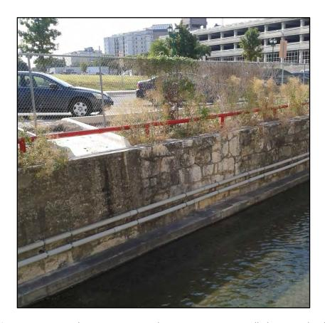
**Figure 4-59**. Seam between stone and concrete retaining wall along east bank.
