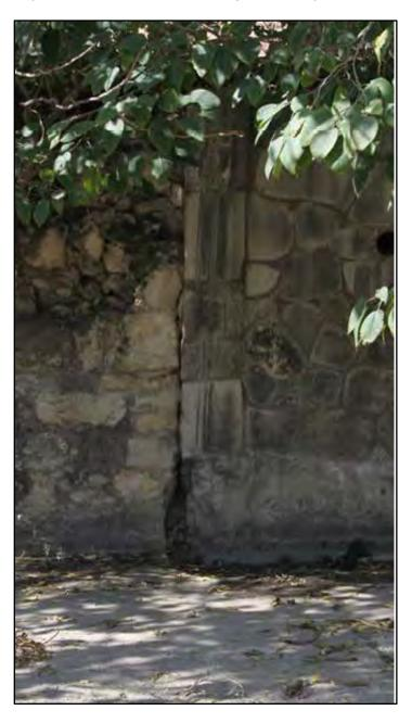
**Figure 4-5**. Joint between two wall segments constructed using different techniques.
