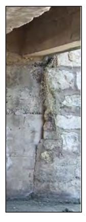
Figure 4-24. Seam at meeting of stone wall and base of bridge at Salinas Street.
