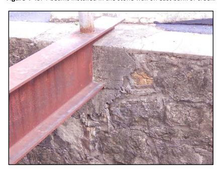
Figure 4-44. Impact to the stone wall resulting from I-beam installation.
