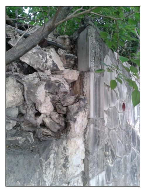
**Figure 4-6**. Close-up of wall joint including the damage suffered by the wall due to root damage.
