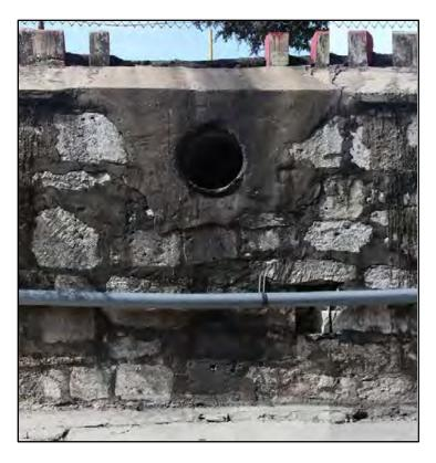
Figure 4-63. Impact to stone wall by drain pipe installation.
