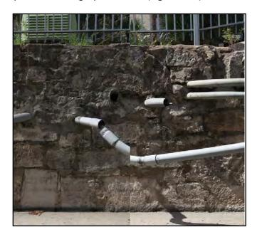
Figure 4-62. Conduits that impact the stone wall immediately south of Nueva Street Bridge.
