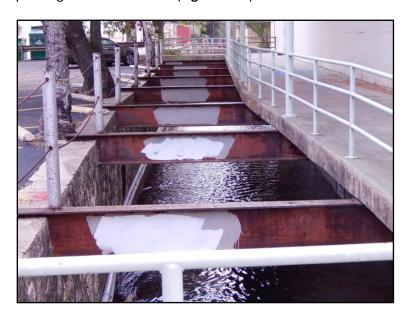
Figure 4-37. I-beams supporting sidewalk along Alameda Theater.
