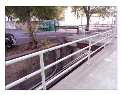
Figure 4-45. Cement revetment covering stone wall between Houston and Commerce Street.
