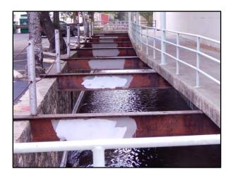
Figure 4-43. I-beams installed in the stone wall on east bank of creek.
