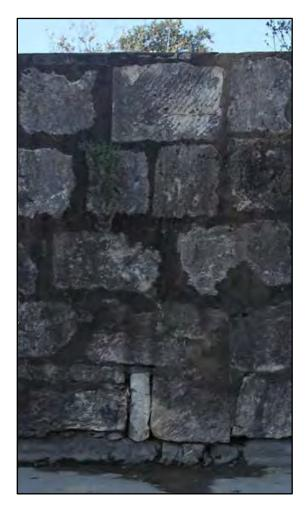
Figure 4-20. Vertical spacers in wall segment just south of Martin Street Bridge.
