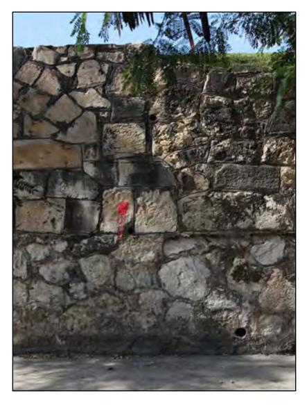
Figure 4-9. Apparent seam in upper stone wall demarcating two distinct construction techniques.
