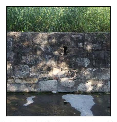
Figure 4-32. Area near base of wall with evidence of construction using recycled materials.
