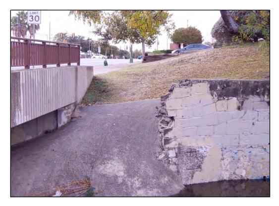
Figure 4-14. Break in stone wall created to allow for construction of Martin Street Bridge.
