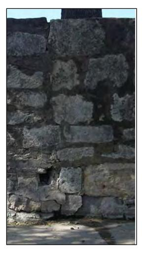
Figure 4-21. Possible seam where construction technique shifts, note drainage hole.
