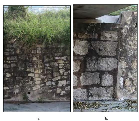
Figure 4-68. Typical stone work in much of this wall segment, note large cut blocks under bridge.
