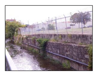
Figure 4-61. Stone retaining wall with concrete wall on top along west bank of creek.
