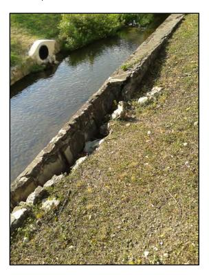
**Figure 4-12**. Erosion of the top of the west bank.
