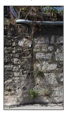
Figure 4-57. Seam between two distinct construction phases or styles along retaining wall.
