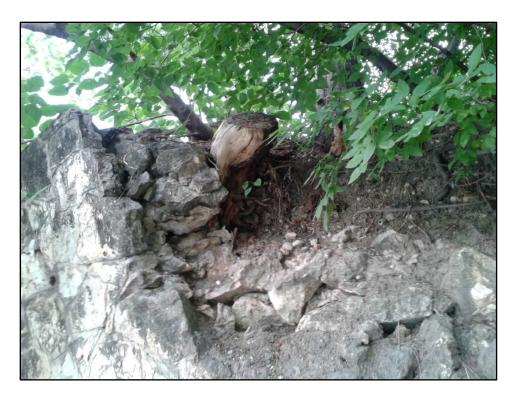
**Figure 4-10**. Inner- and outer-row of rocks that form the retaining wall. Note also the massive damage cause by the roots of the plants growing along the top of the bank adjacent to the wall.
