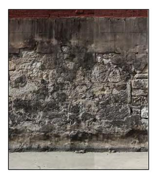
Figure 4-48. Peeling concrete mortar revetment exposing underlying stone wall.
