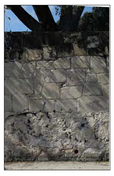
**Figure 4-8**. Smooth faced limestone blocks in upper west wall of San Pedro Creek.
