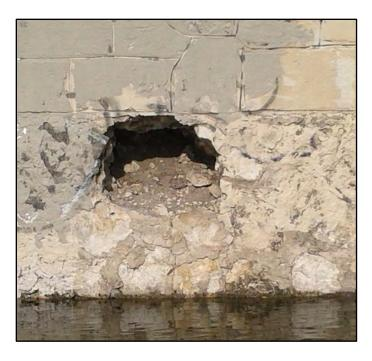
**Figure 4-11**. Large hole developed at the seam between the two wall construction episodes.
