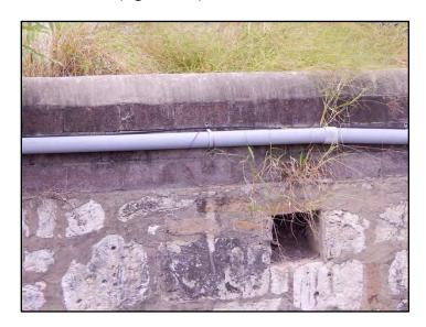
Figure 4-54. Concrete cap on top of stone west retaining wall.
