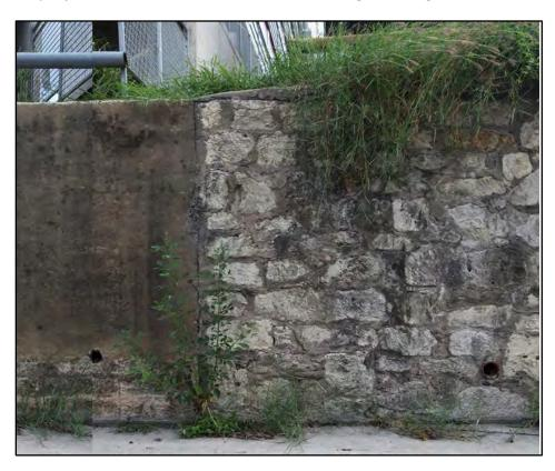
**Figure 4-65**. Elevation of drain pipes in concrete and stone walls of east bank.
