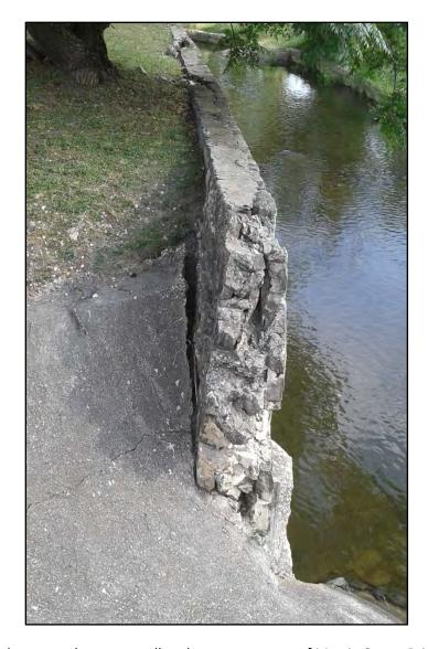
**Figure 4-15**. Gap between the stone wall and concrete apron of Martin Street Bridge, west bank of creek.
