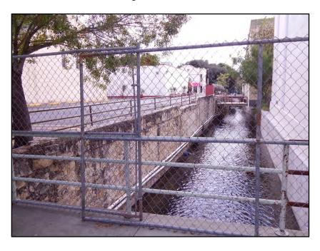
**Figure 4-46**. Stone wall and concrete wall meet along east bank of creek, across from alley between Alameda Theater and the Dollar General Store. Former footbridge was at the seam of the concrete and rock walls.
