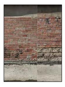
Figure 4-41. Replacement of stone with brick along the Dollar General Store's retaining wall.
