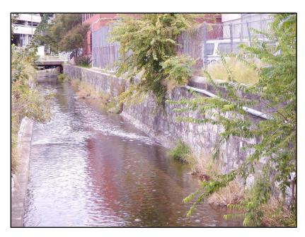
Figure 4-55. Stone retaining wall along west bank of creek, note concrete cap along right edge.
